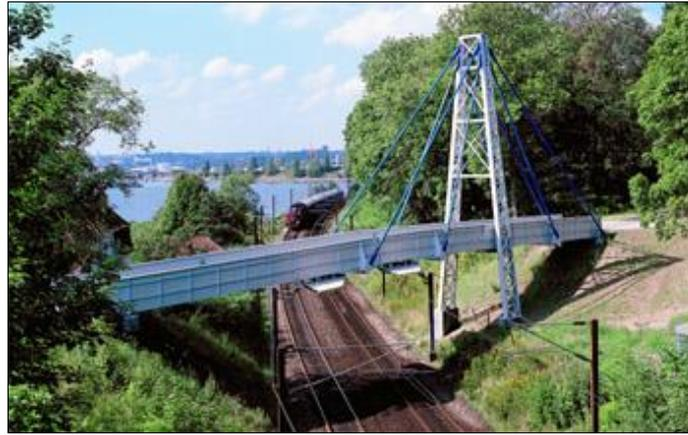
Figure 24 An example of a footbridge made of FRP profiles, there are many similar bridges world wide [27].
