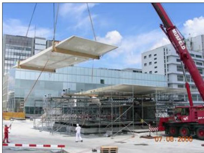
Figure 26 An example of a sandwich structure, Novartis entrance roof, Basel Switzerland [28].
